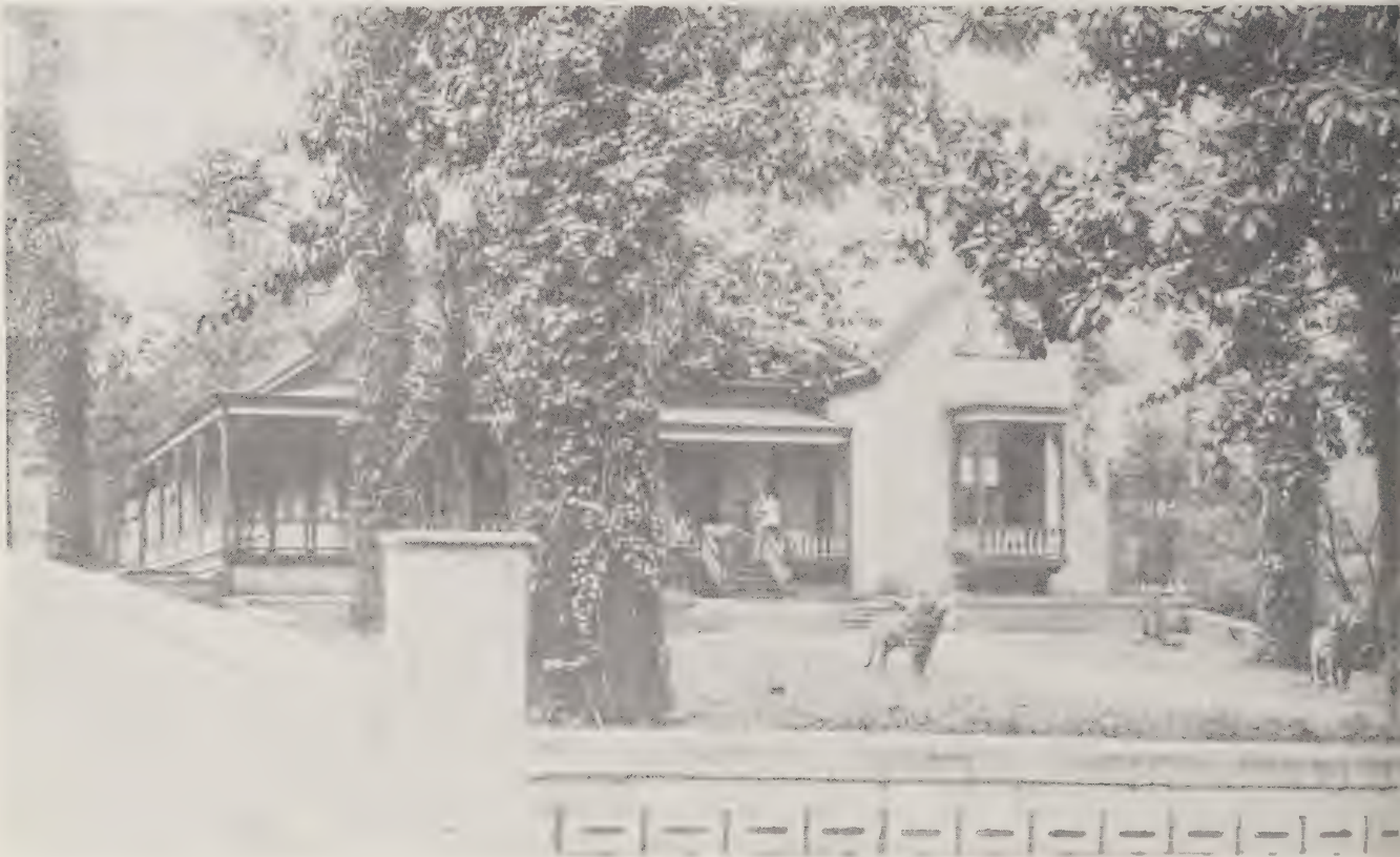
Haas home at the SW corner of McDonough and Alabama Streets has been demolished and is part of Baldwin Junior High School play ground. (1890)
